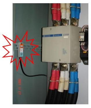
Sensor placement near a Low Voltage Contactor for a Variable Speed Drive
