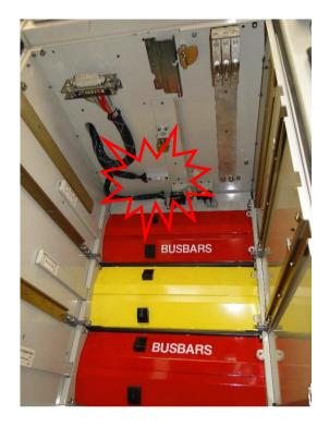
Sensor placement inside the CB racking chamber
