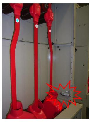
Sensor placement inside the cable termination chamber
