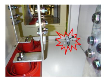
Sensor placement inside the busbar chamber
