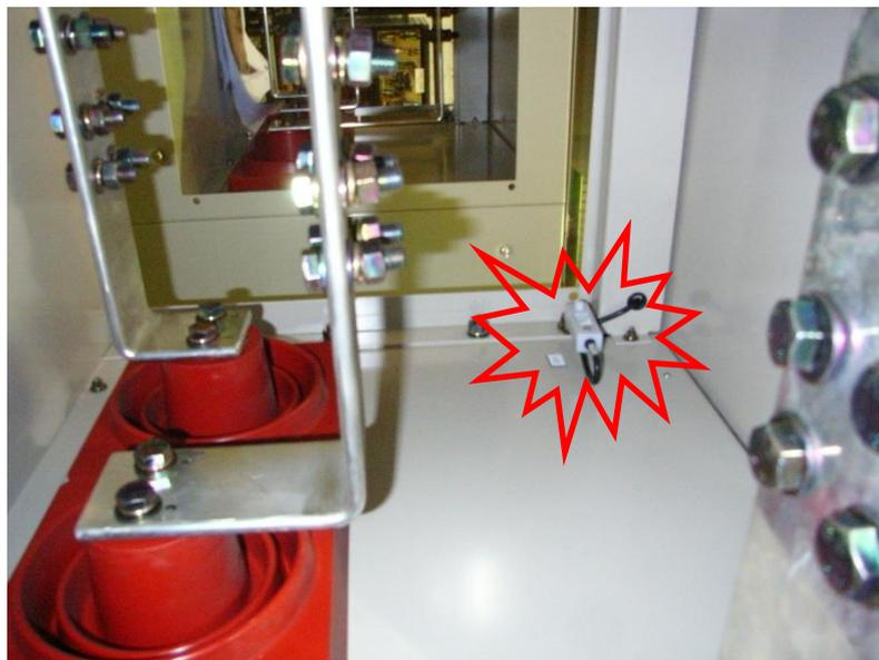
Sensor placement inside busbar chamber
