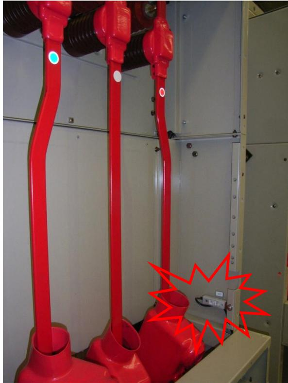
Sensor placement inside cable termination chamber
