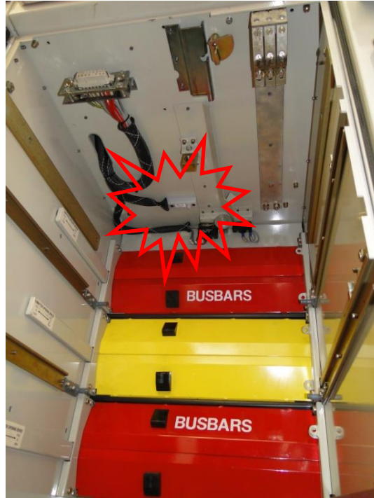
Sensor placement inside CB racking chamber
