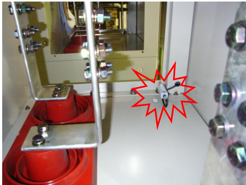
Sensor placement inside busbar chamber
