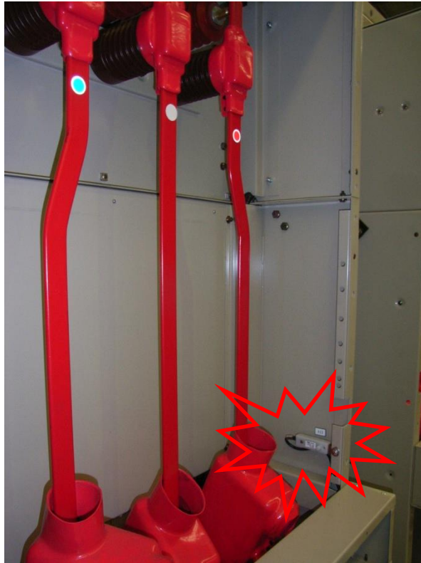
Sensor placement inside cable termination chamber
