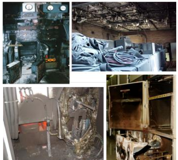
Figure 4: Consequences of arcing faults
